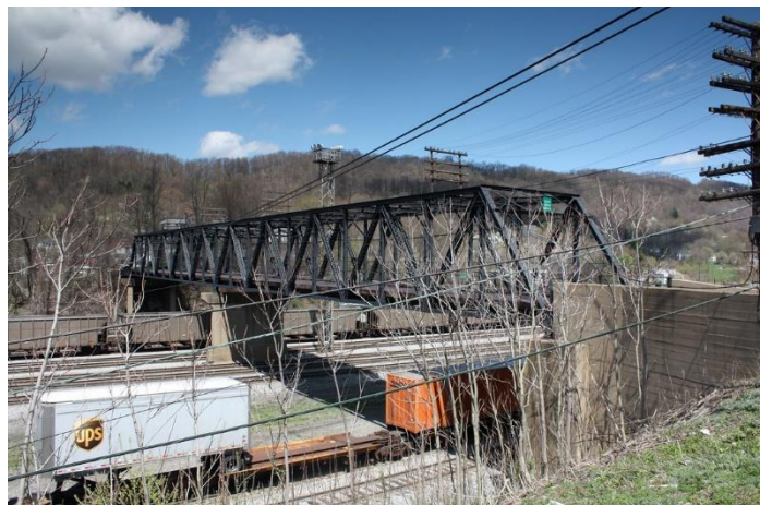
Figure 33 - Truss Bridge in Bluefield, WV
